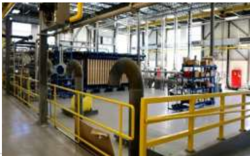
City of YK Water Treatment Plant. Source: myyellowknifelow.com
